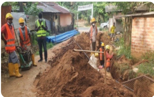
Walapane Pipe laying
