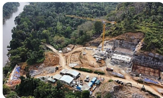
Water Treatment Plant and Intake
