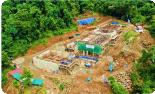
Construction of Water Treatment Plant
