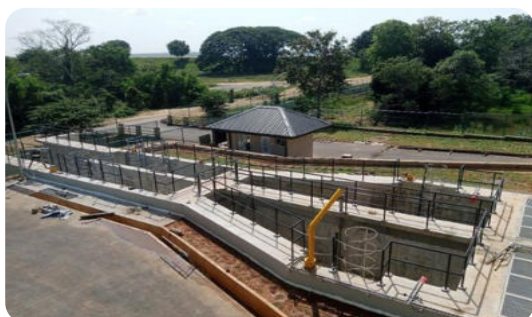
Mahakanadarawa Water Treatment Plant Intake
