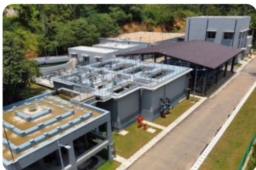
9000 m3 water treatment plant Ukuwela
