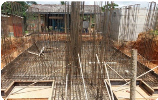
Flocculator & Sedimentation Tank of the Hallala WSP Stage I
