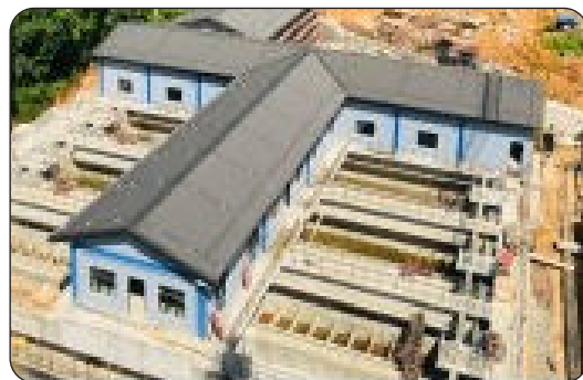
Water Treatment Plant – Karasnagala
