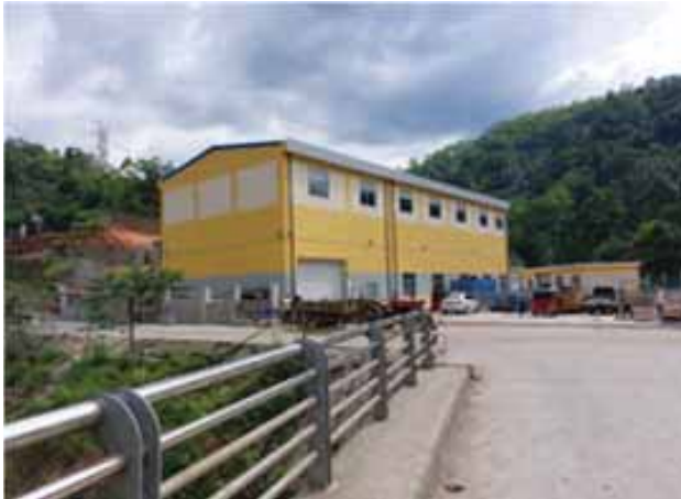
Figure P4: Broadlands power house building
