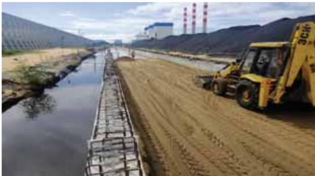
Figure G4: Coal yard extension works in progress
