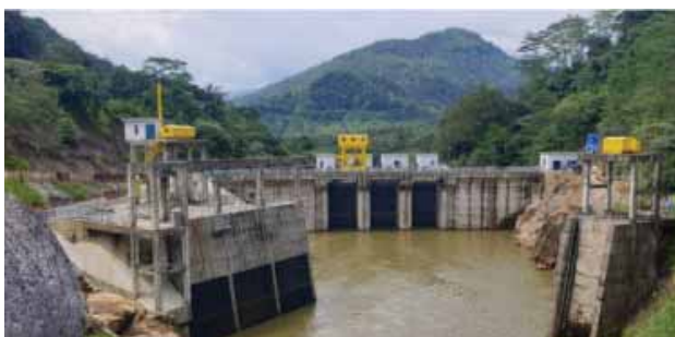
Figure P3: Broadlands main dam and the reservoir
