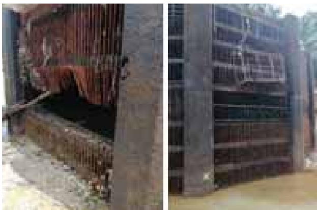
Figure G1: Intake screen before and after the repair
