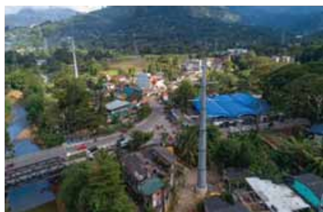
Figure P6: Erected monopole tower under Uma Oya Project
