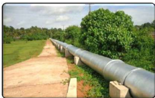
1000/ 800 DI Transmission Main from Bandaragama to Piliyandala (Package 2)
