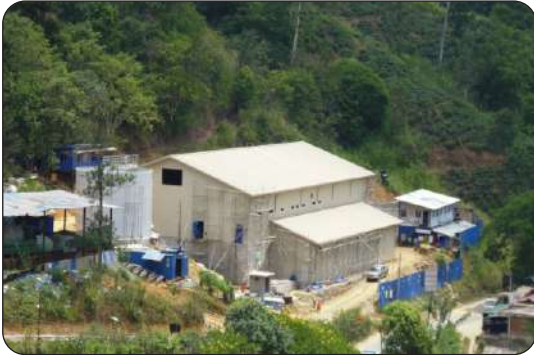
Labugama Water Treatment Plant
