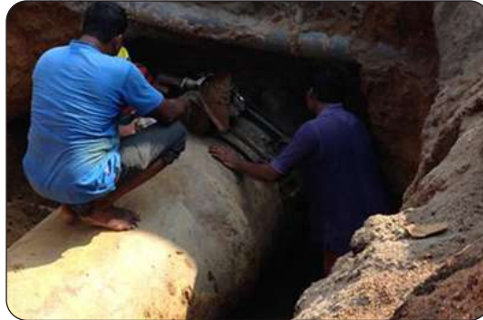
Biyagama - Mabima pipe laying work
