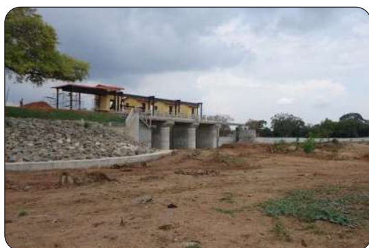
Spillway Structure NeroPer-Aru Dam construction in Vavuniya
