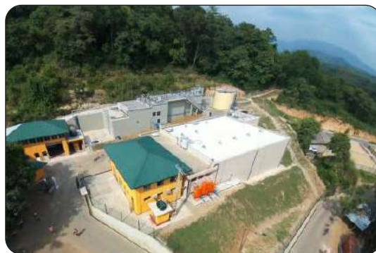
Kumbukkana treatment plant
