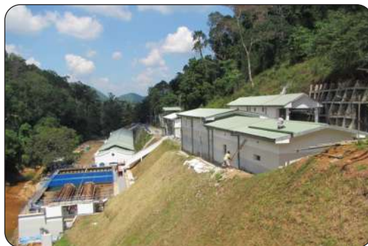
Construction of water treatment plant at Demodara
