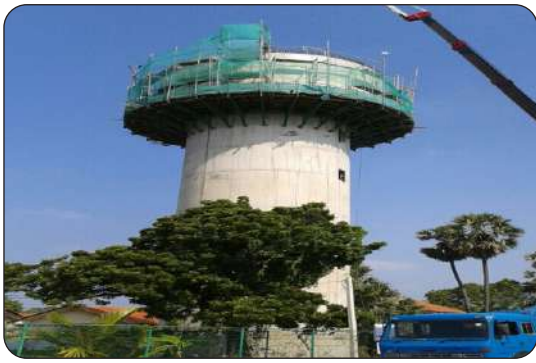
Water Tower at Velanai
