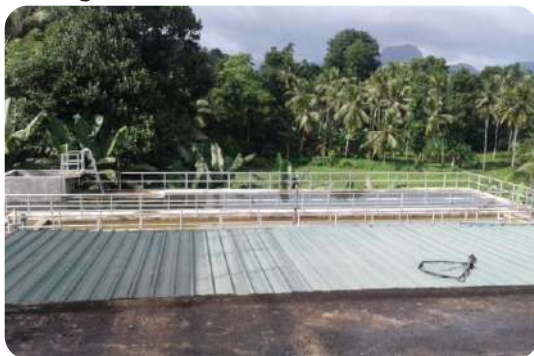
Mawanella treatment plant
