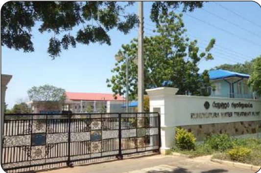
Ruhunupura Water Treatment plant
