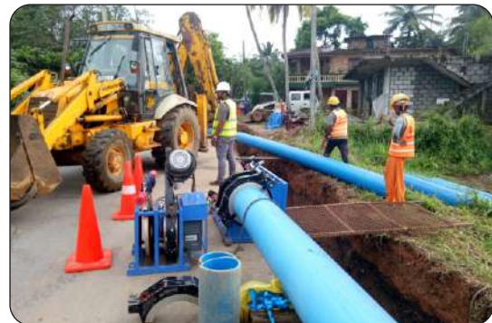
Preparation for 355mm dia pipe welding at Meegoda-Dampe Road
