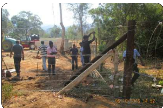
Elephant fence arranged for Contractor's main yard
