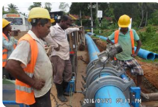
Pipe laying at Baddegama Hikkaduwa High way access road
