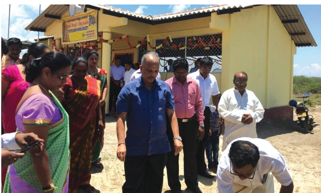
Construction of a Cultural Centre at Sivapuram, Thiruketheeswaram, Mannar by the People's Bank Hindu Society.
