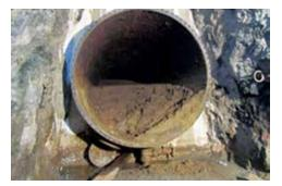
Silt deposited in the steel liner at Adit No. 1
