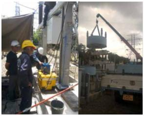
Circuit Breaker Testing at Ampara GS
